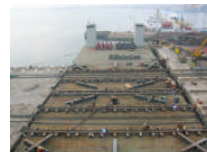
Support steel on bank of the vessel
